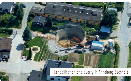
Sealing a mine shaft
