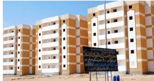
Fig.15: Vacant housing units in a new city
