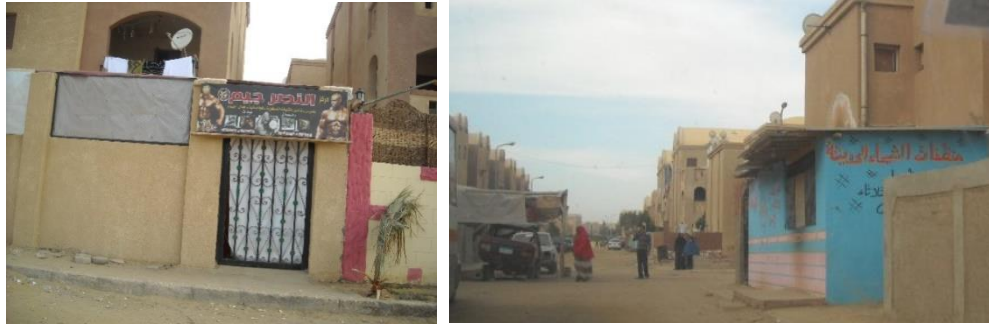
Figure 3 Appropriation of ground floor at Haram City, Source: Author
